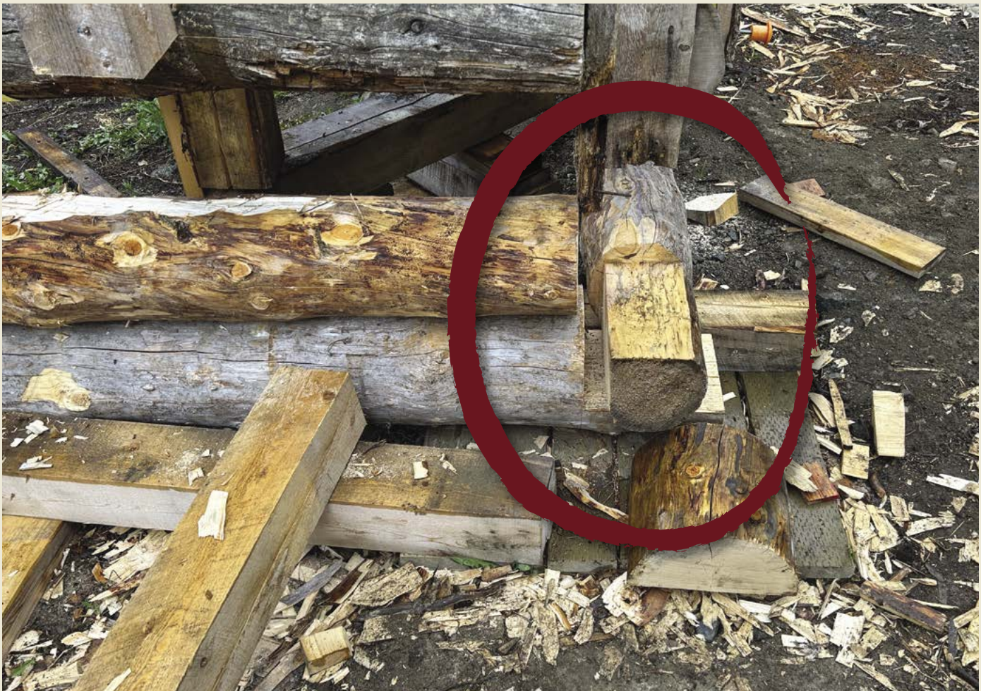
Cabin 1, northeast corner, square lapped corner, see 'Log Building Corners' poster on page 4.
