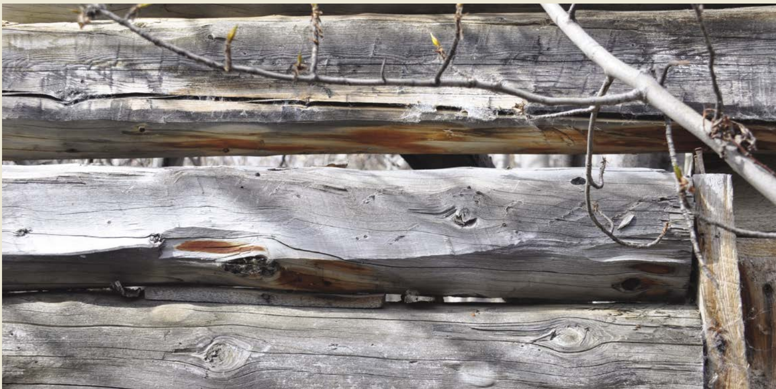
Cabin 1. Axe - hewing techniques on three logs.
