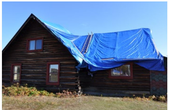
Stone House roof repairs
