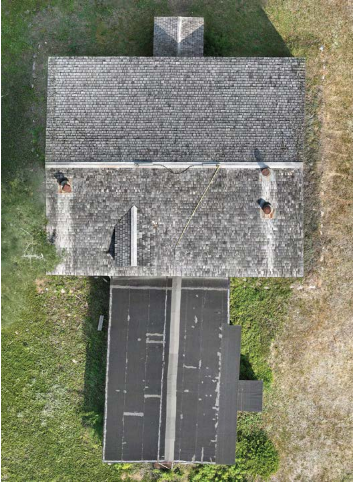
▲ Anglican Rectory roof before.
