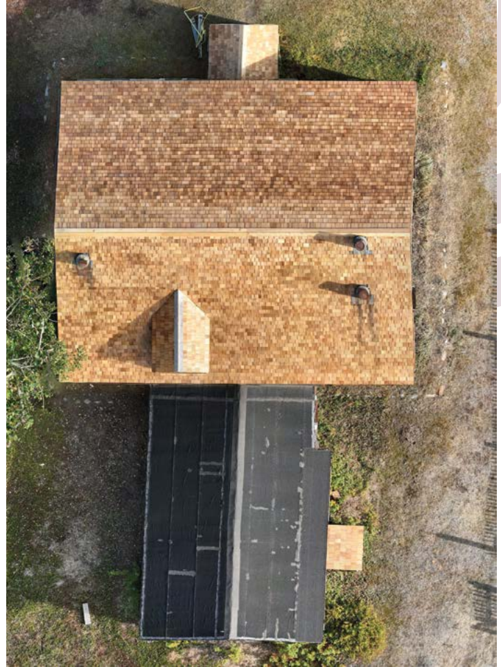
▲ Anglican Rectory roof after.
