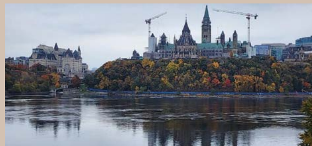
Photo from L-R: Fairmont Chateau Laurier, where the National Trust Conference was held, Rideau Canal locks and the conservation work being done at the Parliament building. Photo taken by Sean McDougall across the Ottawa River from the grounds of the Canadian Museum of History.
