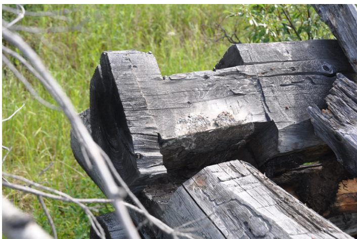
LaPierre building corner joint detail, 2012.
