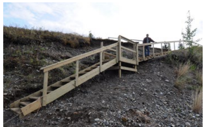
New stairs up from the river to the site.
