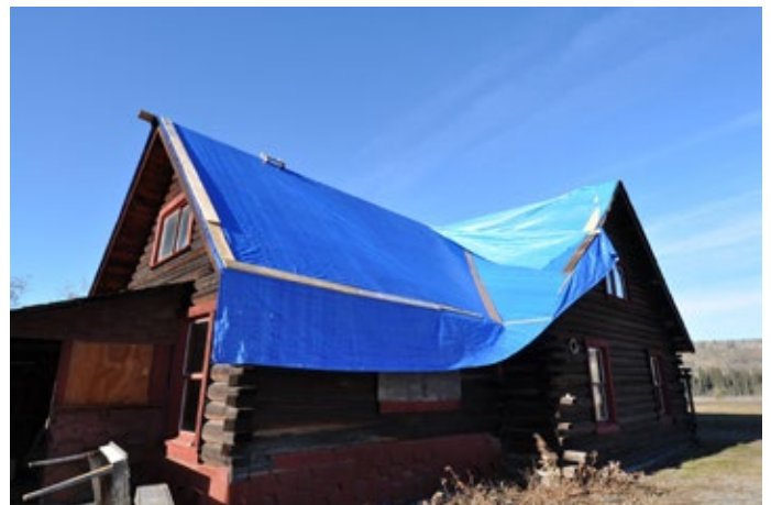
Stone House tarped at the end of the 2018 work season.
