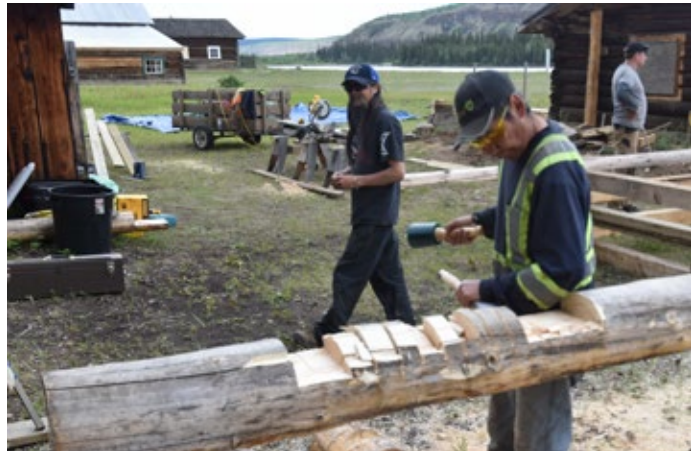
Sill log being notched for door.
