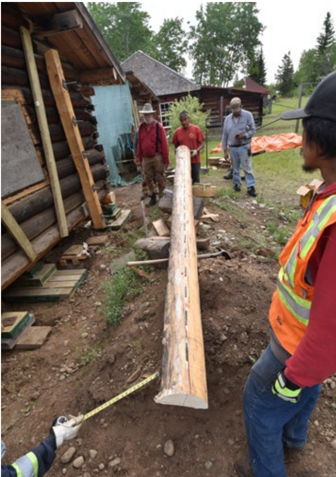
Sill log ready for installation.
