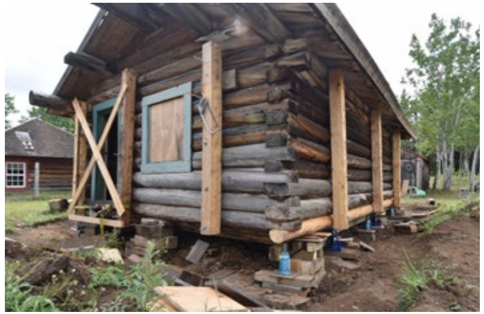
Devore cabin lifted, new sill logs being added.
