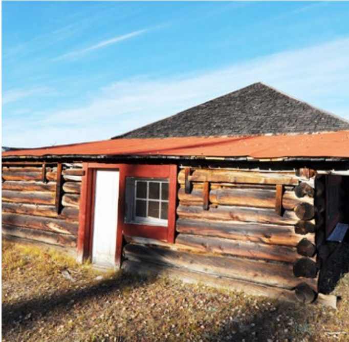
R.C.M.P. Building with new shed addition roofing.
