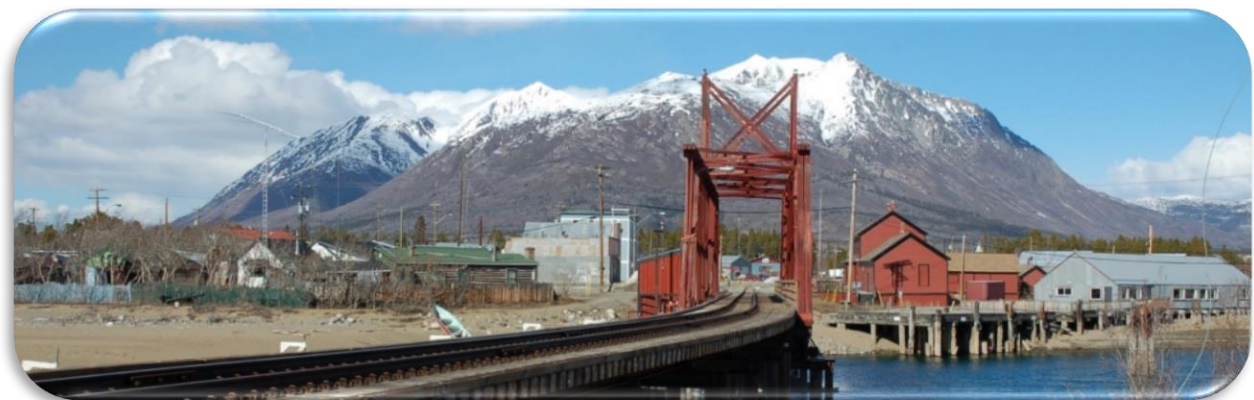
Panorama view captures downtown building and bridge scale in mountain landscape context
