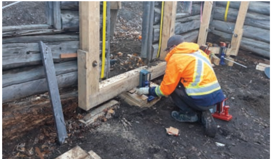
Approximately 18" lift on the highest corner.
