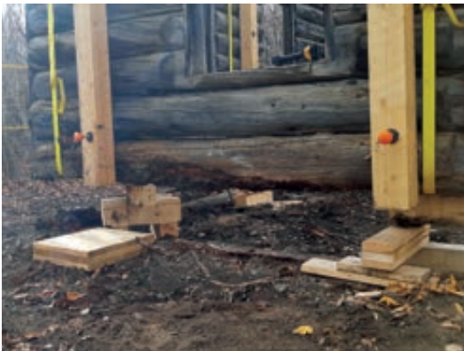
Interior view of SW corner, after lift. Sandwich bracing with cribbing in place.
