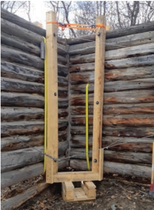
Interior view of SW corner, after lift. Sandwich bracing with cribbing in place.
