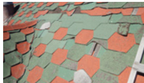
▲ Stone House roof shingles - Before
